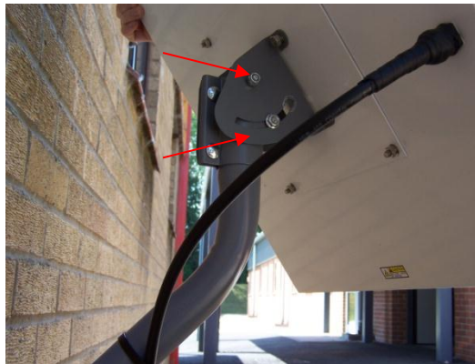
Figure 4-13 - Adjusting elevation
